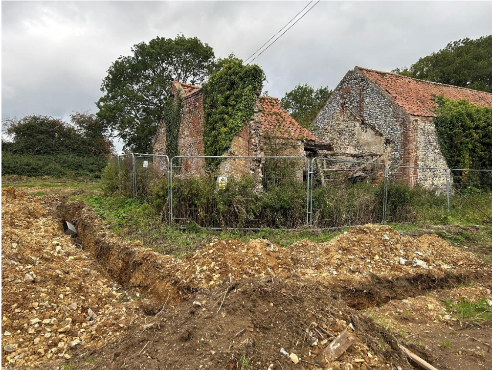
Plate 12-6 Derelict property at Abstraction 6/33/58/*G/0248
