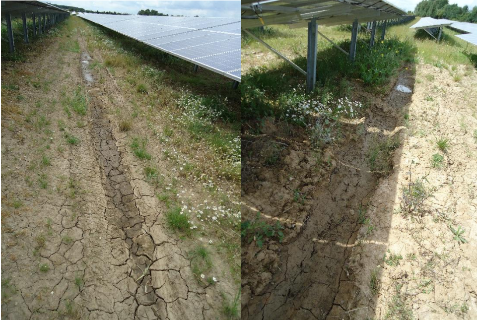
Plate 12-21: Poor practice vegetation establishment examples on solar sites
